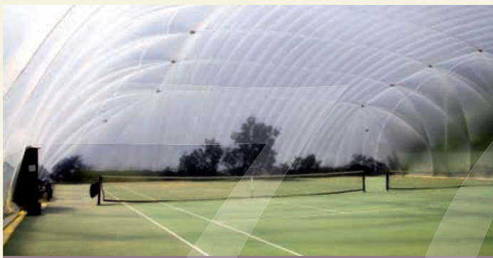
Covered flood lit courts
